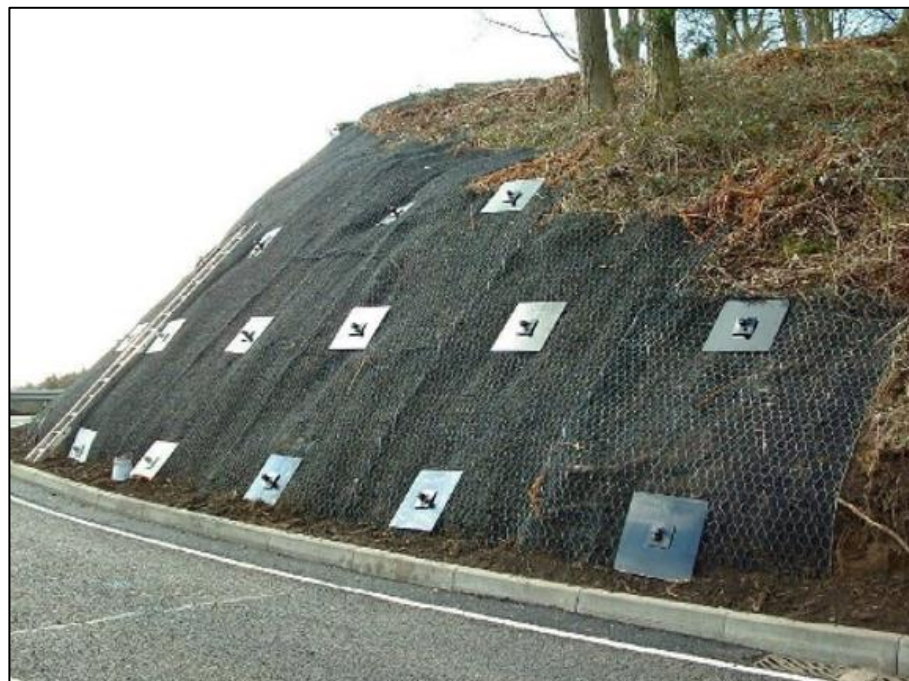
Fig 1: Soil Nailing
